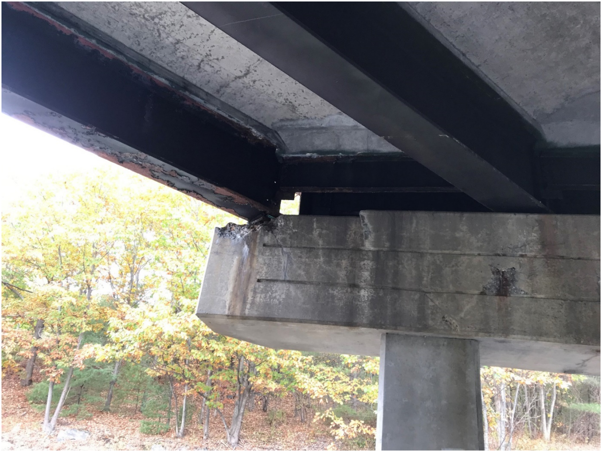
Southbound fascia and pier cap spalling at fascia beam
