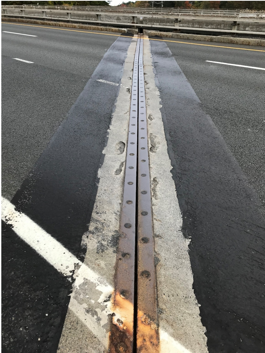
Southbound expansion joint at pier
