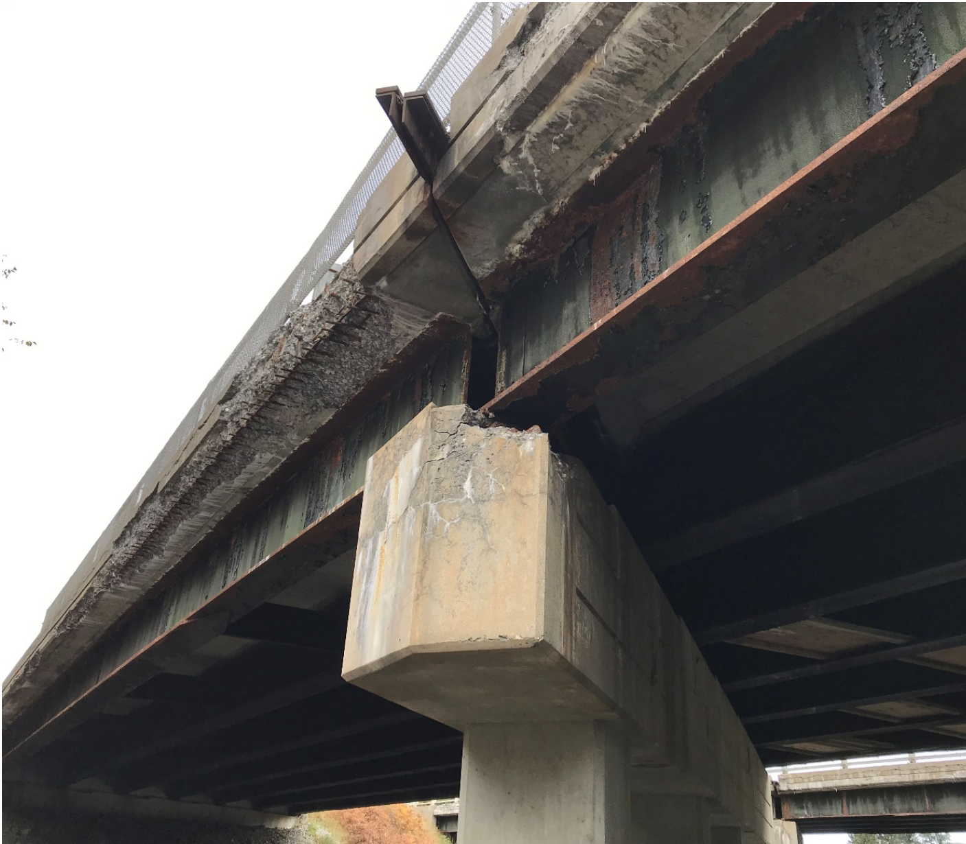
Southbound fascia and pier cap spalling at fascia beam
