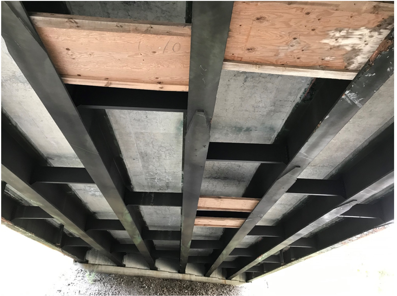
Typical condition of underside of deck
